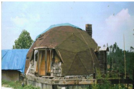
Figure 2.12: A dome house hit by an EF5 tornado in West Jefferson County 1998 (AGE dome)
