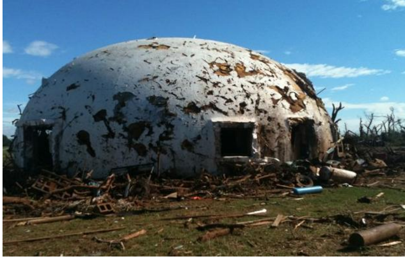
Figure 2.8: A dome hit by a tornado on May 24, 2011 in Blanchard, OK (Josh South)
